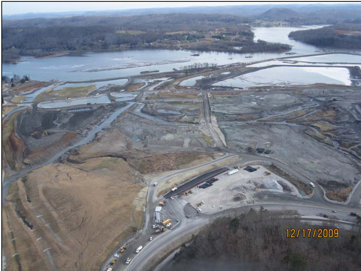
Photo shows Swan Pond Embayment and failed dredge cell.
